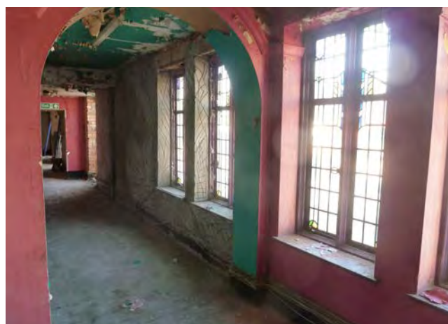
Internal corridor, front building, 2016
