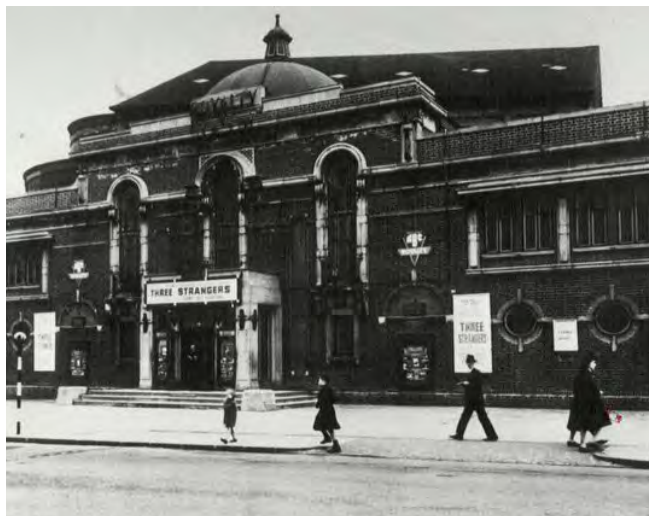
1941 photograph of the Royalty Harborne. Source unknown. Note the Cupola above the dome was removed prior to the 2015 survey.
